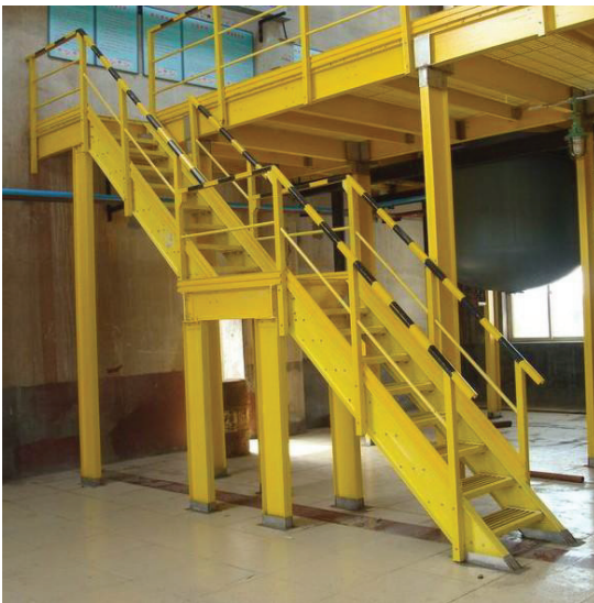
FRP Handrails and steps in Chemical Factory
